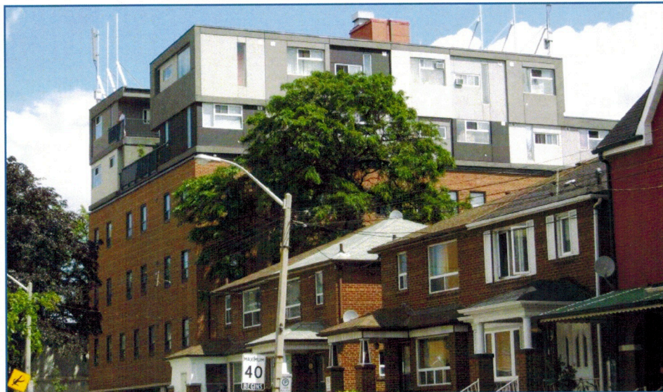
Figure 1 St. Clare's first housing project was the conversion of a medical building at 25 Leonard Avenue, now affordable housing with 77 units.
