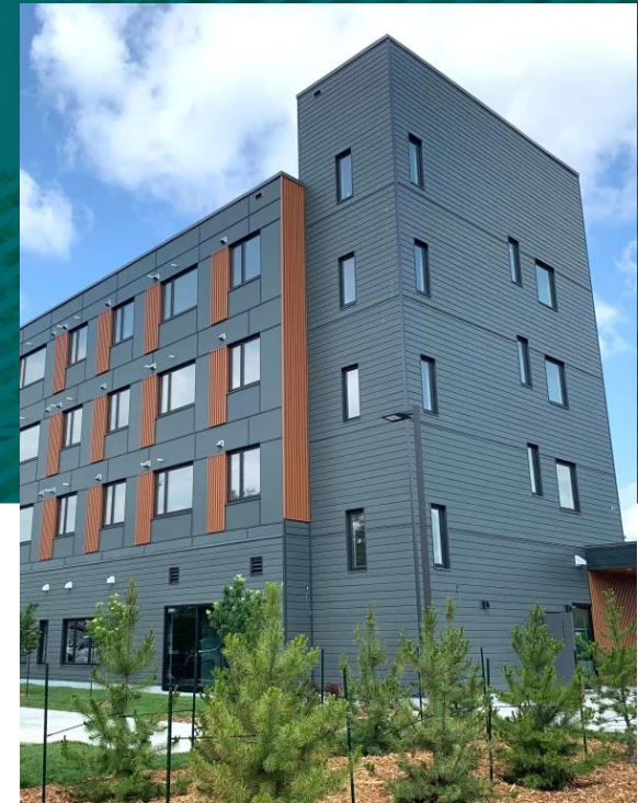
Doing the work
